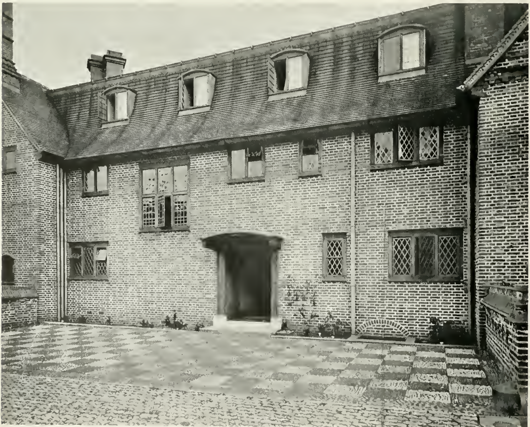
BISHOPSBARNS, YORK: VIEW OF THE NORTH FRONT. WALLS OF HAND-MADE BRICKS, AND WINDOW-FRAMES OF ENGLISH OAK; A TILED ROOF, AND A FORECOURT PAVED WITH BLACK AND WHITE PEBBLES
